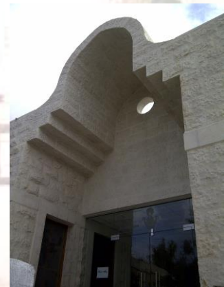
Fig. 29 Administration Building Entrance.
