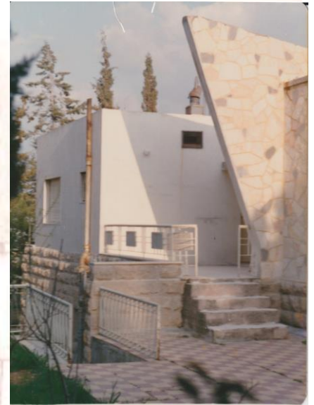
Fig. 21 Existing Shear wall
