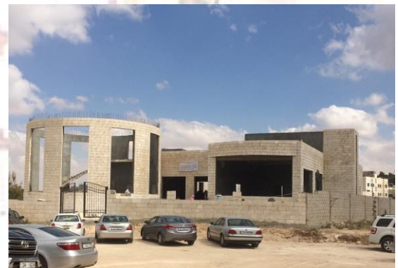
Fig. 46 Building during construction
