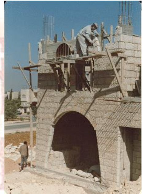
Fig. 13 Villa Construction at Basement level.
